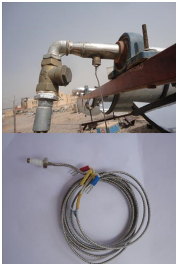
Fig (7) Thermometer (thermocouple), anti-return valve
